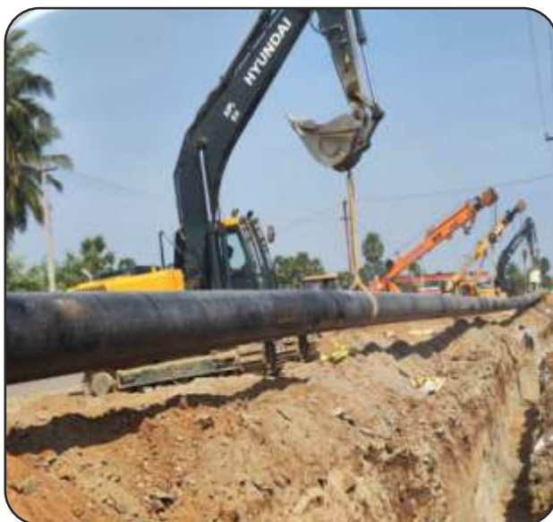
Lowering in Progress
